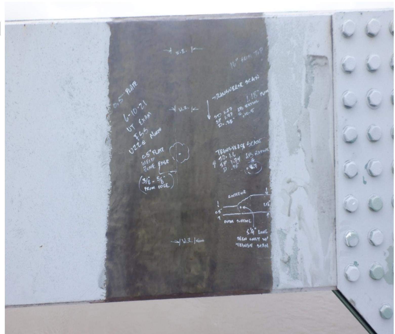
NDT Inspection of Arch Rib Member
