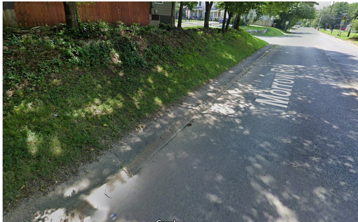
Morrow Rd rebuild
