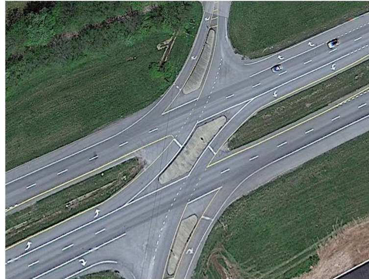
State Route 6 at South Cross Bridge Road
