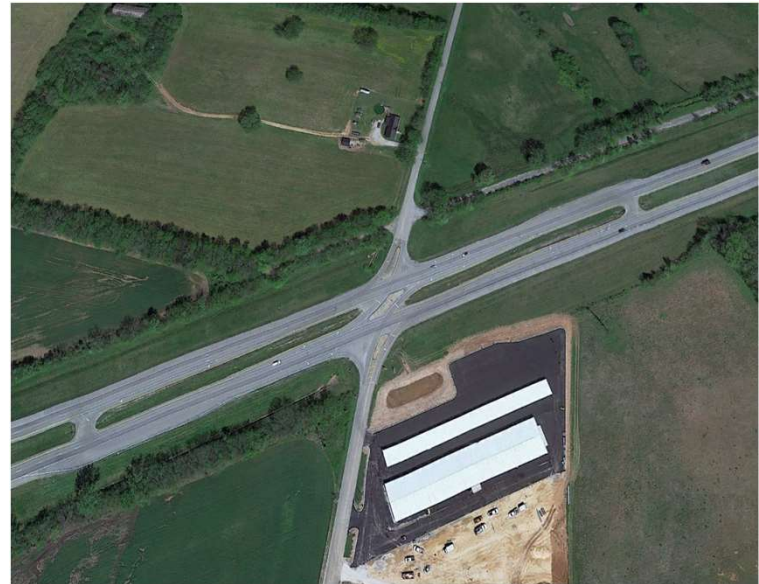
State Route 6 at South Cross Bridge Road
