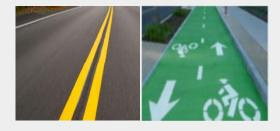
**Transverse markings** are generally placed perpendicular or across the flow of traffic. They help define important roadway features such as intersections and crosswalks. Examples include stop lines, turn arrows, and word markings.
