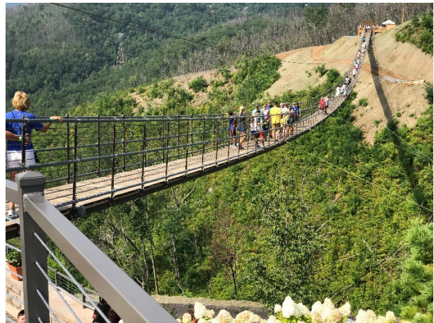
Picture 5: Skybridge Gatlinburg Technical Tour
